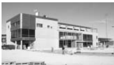
Fig 1. View of one of the buildings.
